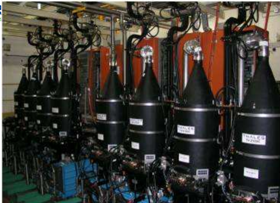
TH2013C: 700kW CW on matched load
